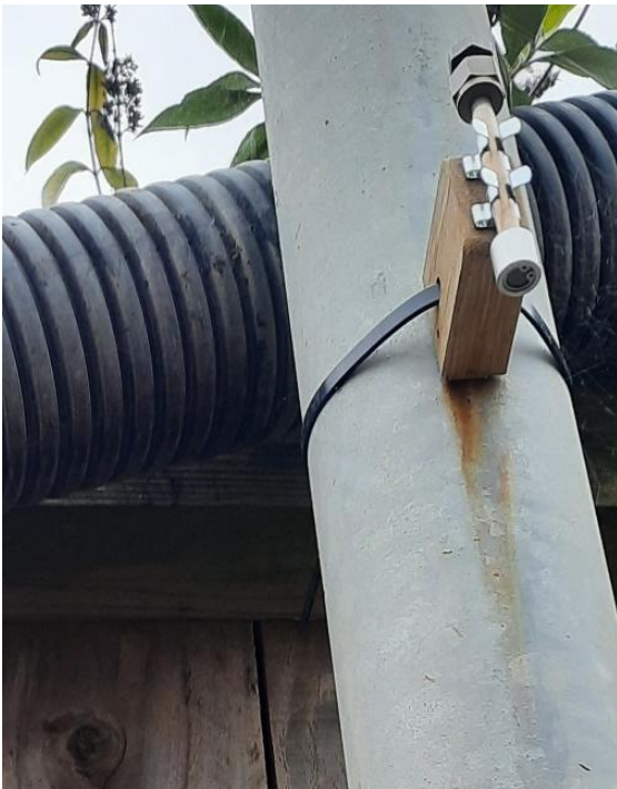
Photo 4.1 – Passive (diffusive) Tenax tube monitoring (Note how the tube is held vertically by clip, away from interferences, with a dust cap on the end).
