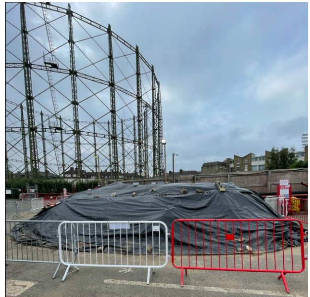
Photo 8.2 – Covering over stockpiles of residual odorous material is good practice
