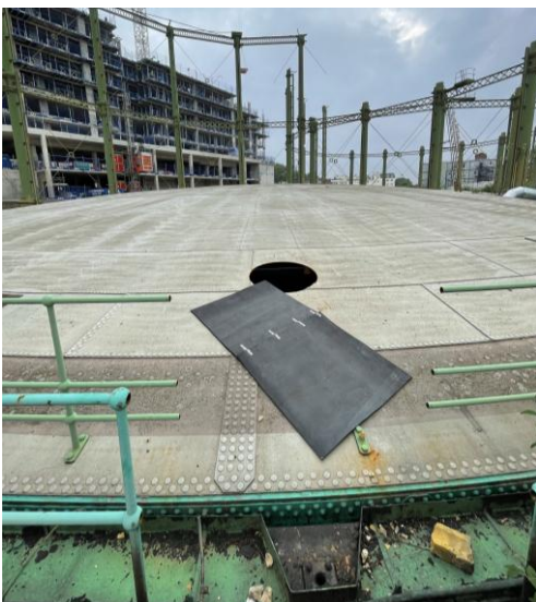
Small aperture in gasholder crown
